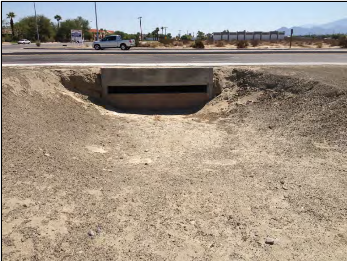
Exhibit 6-1 Existing Concrete Culvert
